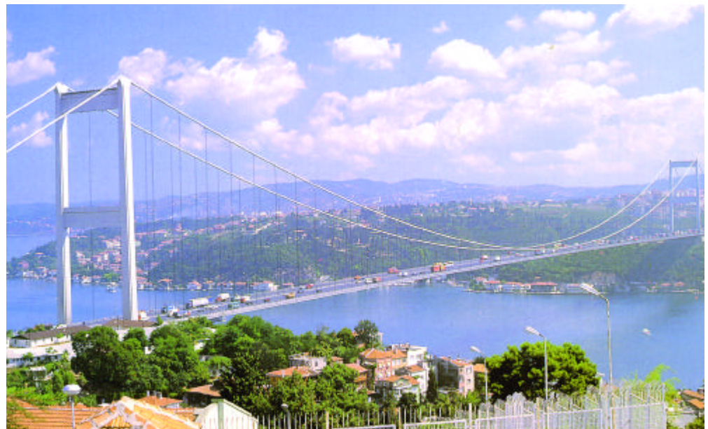
Bosphorus Bridge in Istanbul
