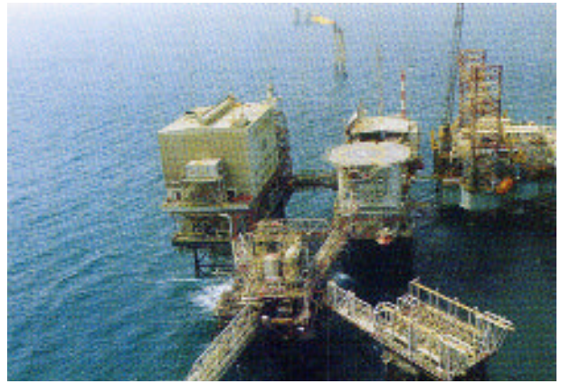
North Gas Field
